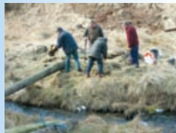
Bridge-building near Balgothrie
